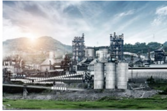
Building materials transport of cement required pressure 4 bar
